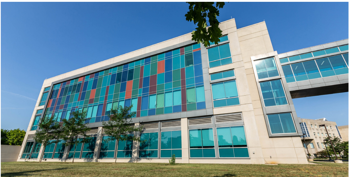
Science and Engineering Laboratory Building IUPUI Campus
